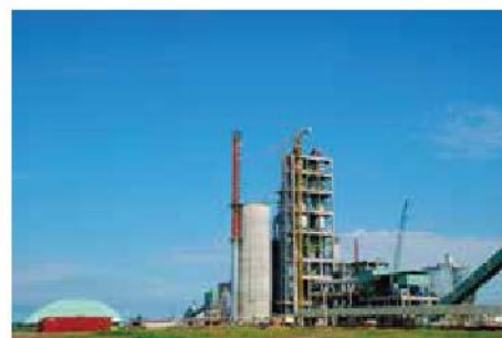
Binh Phuoc Cement Plant
